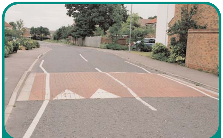
3.1 Flat topped road hump with a short plateau as it is not on a bus route
