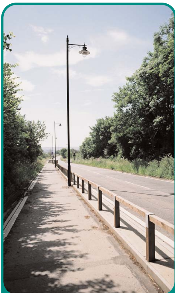
2.2.1. Segregated facilities for cyclists, pedestrians and horses beside a bypassed road - reallocation of the road space.
